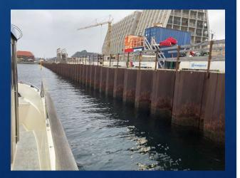
At vertical structures the system is more challenged by multipath. A normal *Bottom* Detection Algorithm is then not adequate. We need something else for these cases.
